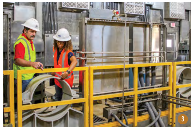
1: GCWA reused existing vertical turbine pumps for the new 96-MGD pump station. 2: The project was divided into four phases to ensure the new pump station was up and running as quickly as possible. 3: Custom-designed carbon steel pipe was installed to support future above-grade pump discharge piping. 4: Three new eight-foot-wide traveling screens were installed as part of the new intake structure.
