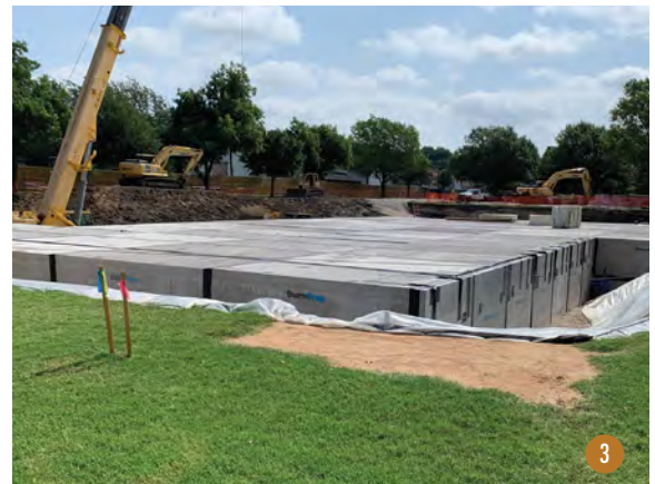
1: Phase one installation of StormTrap—only a small crane was needed on-site to lift individual precast pieces into place. 2: Huitt-Zollars and City of University Park personnel inside installed modular system. 3: Installation of phase one nearing completion.
