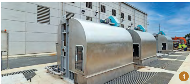
1: GCWA reused existing vertical turbine pumps for the new 96-MGD pump station. 2: The project was divided into four phases to ensure the new pump station was up and running as quickly as possible. 3: Custom-designed carbon steel pipe was installed to support future above-grade pump discharge piping. 4: Three new eight-foot-wide traveling screens were installed as part of the new intake structure.
